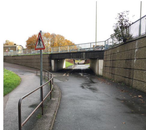
Paving in southern underpass
