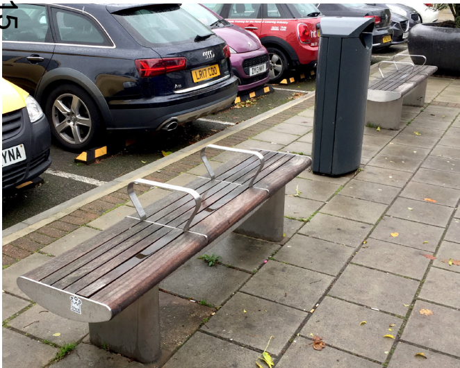
Existing timber and stainless steel benches and powder coated steel litter bin suitable for reinstatement as part of the new furniture palette, after cleaning up, assessment of their conditions and refurbishment when necessary.
